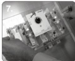
7. Install fuse shroud into the corresponding clips
